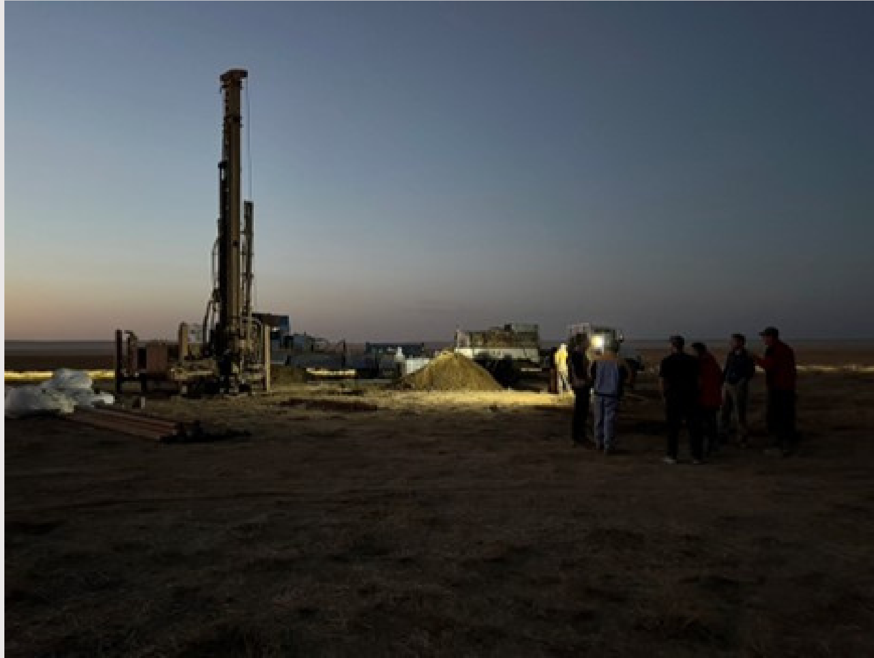
Waterwell rig at UNWH-01, Urgakh Naran.
